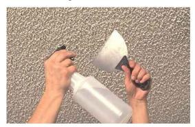
I can't stress enough how important it is to treat your popcorn ceiling as though it contains asbestos until analysis by an independent laboratory proves otherwise. Don't get the notion that today you are going to scrape the popcorn off the ceiling. Stop and think about the consequences before you begin. This individual is ready to dive into a project but is not wearing protective clothing or gloves. Even taking a small sample requires protective measures!
