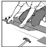
**[7]** It's easier to assemble if you kneel on top of the planks and use a pulling motion to insert.
